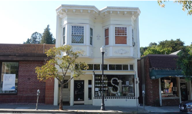
Example of Main Street Building
