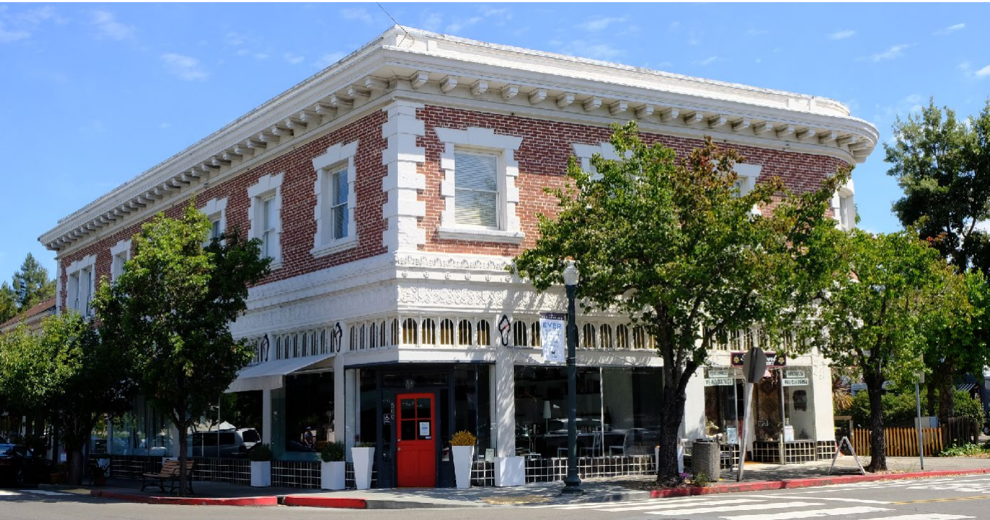
Example of Main Street Building
